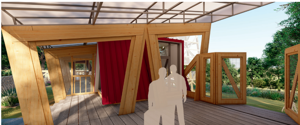
Figure 10. The porch's main section consists of wood-sandwich space trusses topped by a metal awning frame supporting a stretched fabric canopy.
