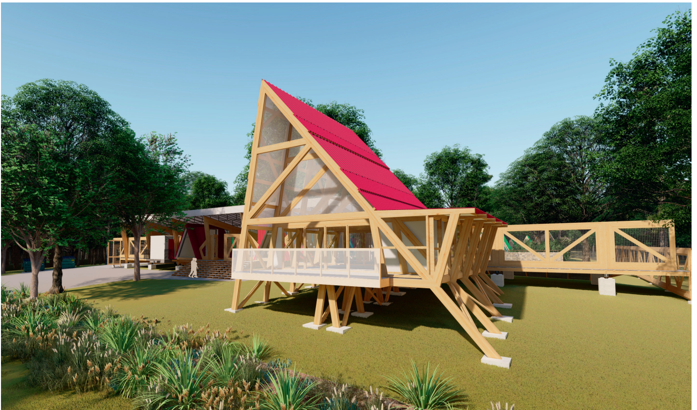
Figure 13. The community hall's asymmetrical A-frame is responsive to different edge conditions and solar orientations.
